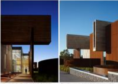
Use of local, reclaimed and recycled materials - Photo Credit: Kate Joyce Studios
